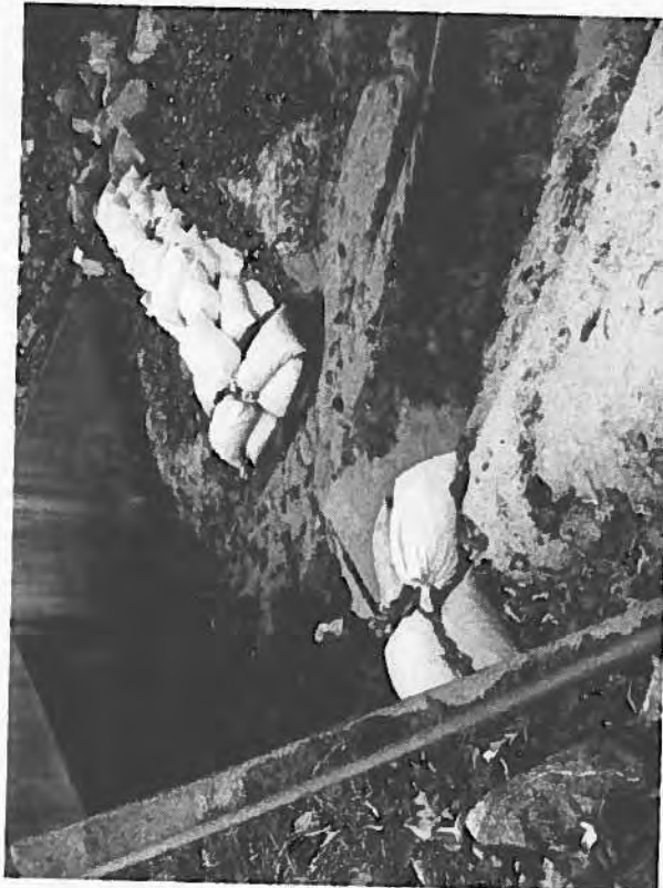
Ongoing attempts by St. Martin's Church to manage the sediment load they receive from unmanaged stormwater flows upstream in Winston Terrace and Colony Sq Shopping Center. Sediment blocks downstream flow and causes flooding in church facilities.
